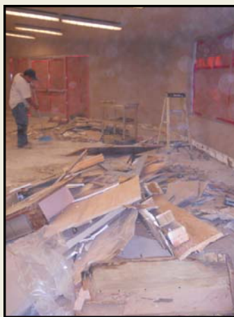
Crews quickly demolished the Meerkat Café.
